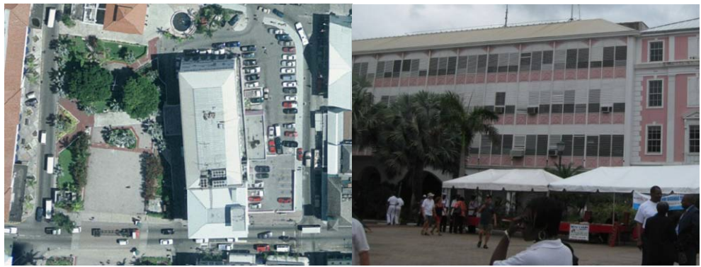
Figure 3-6: Aerial view and front view of the Cabinet Office
