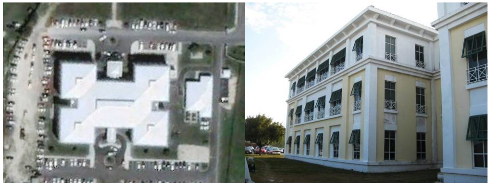
Figure 3-12: Aerial view and front view of the Ministry of Education
