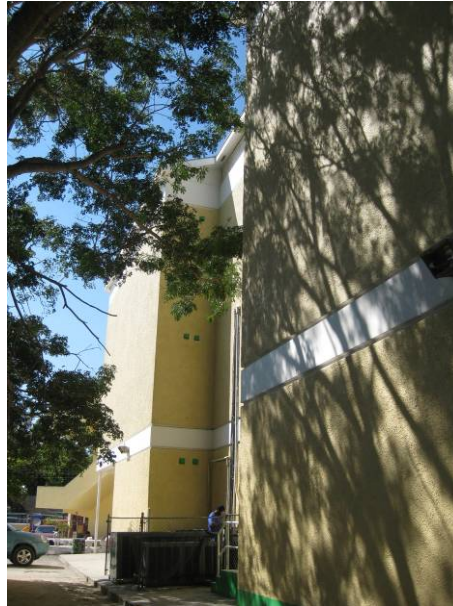
Figure 3-22: "Light coloured school building shaded by a tree"
