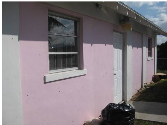
Figure 3-21: "Light coloured office building with partial shading by eaves"
