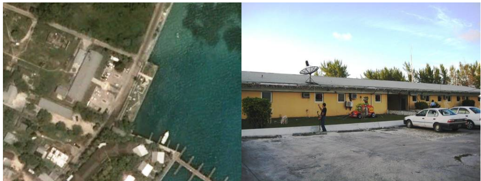
Figure 3-14: Aerial View and front view of the Bimini Administration Building
