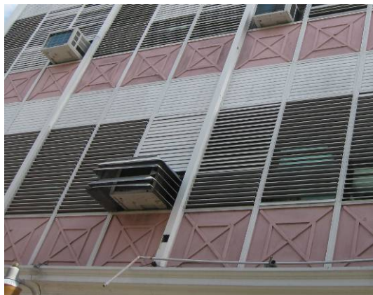
Figure 3-23 "Building with hurricane shutters and shaded decentralized A/C system"
