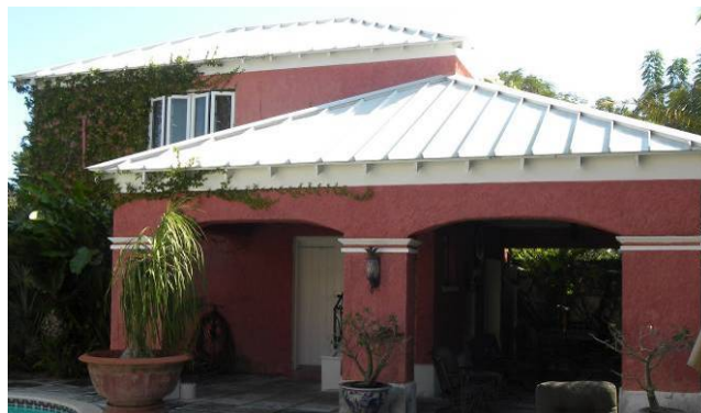
Figure 3-45: Light colored and reflecting roof but dark and absorbing walls
