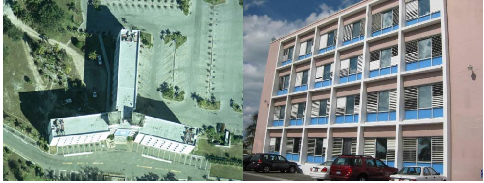
Figure 3-5: Aerial view and front view of the Ministry of Works & Transport
