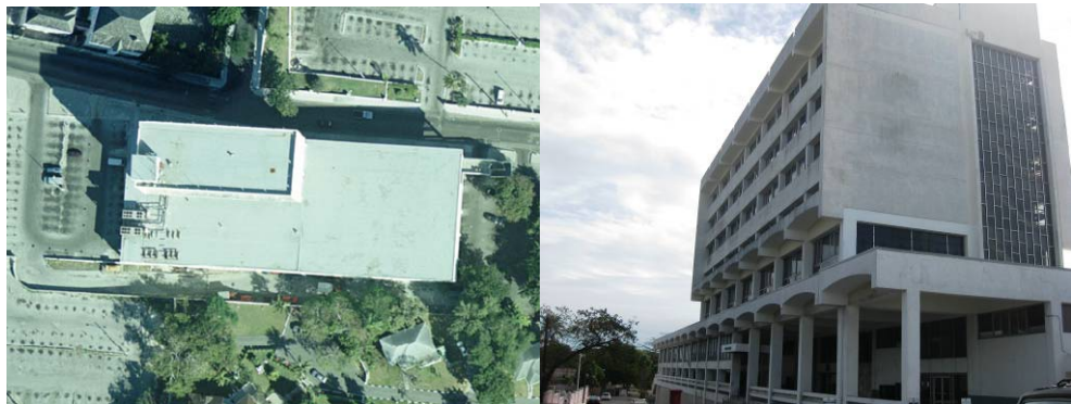
Figure 3-8: Aerial view and front view of the Main Post Office
