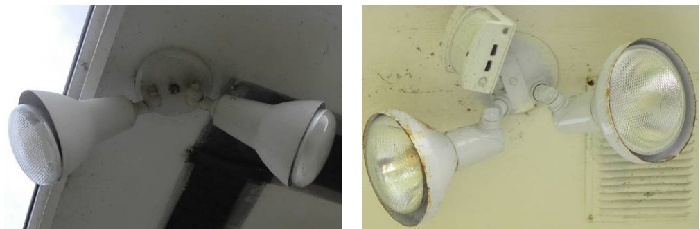
Figure 3-46: Security lights without (l) and with motion detector (r)
