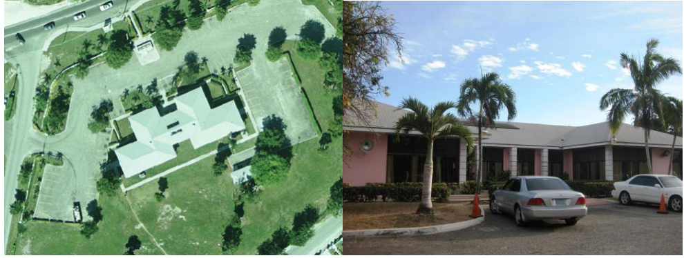
Figure 3-9: Aerial view and front view of the Elisabeth Estate Clinic
